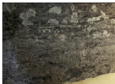
The unreinforced concrete walls before FRCM treatment.
