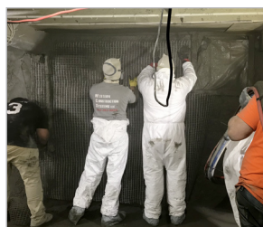
Preparing carbon grid for second layer of cementitious matrix.
