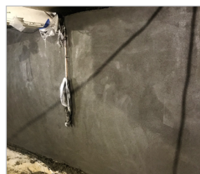
The final surface of the FRCM with a trowel finish.
