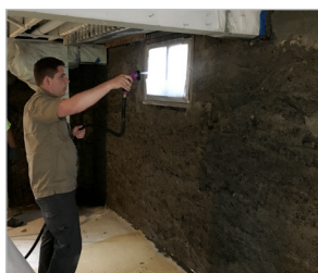
Spray-applying water to the concrete to create a saturated surface-dry (SSD) condition for the cementitious matrix (CSS-CM) installation.
