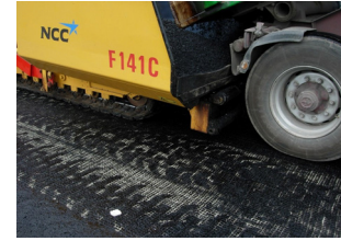
2006 — Asphalt layer being installed on top of asphalt reinforcement grid.
