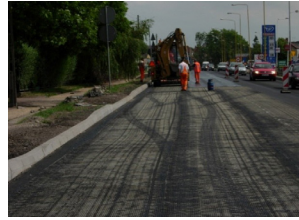
2006 — Asphalt reinforcement grid installed.
