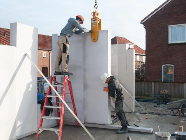
Installation of AAC wall panels
