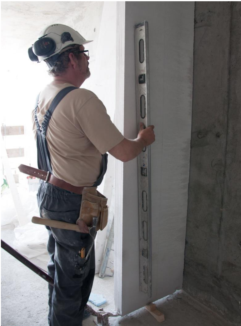
Level the panel vertical and horizontal
