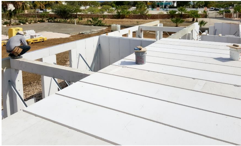
Installation of floor/roof panels
