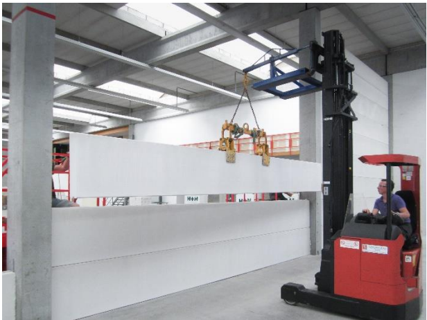
Installation of industrial wall panels
