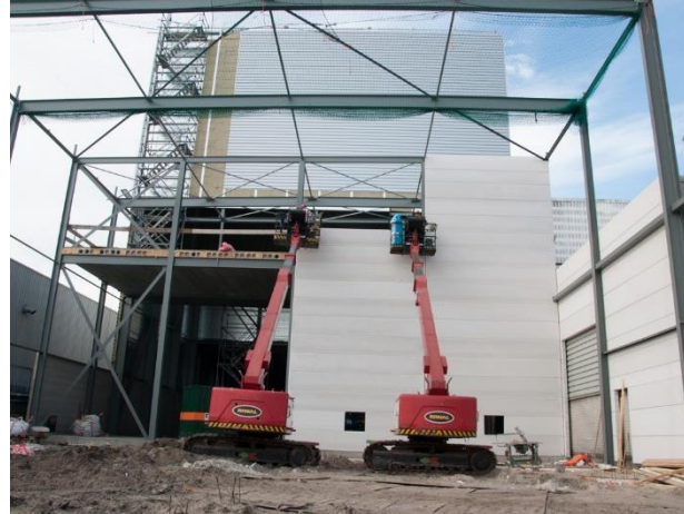
Installation of industrial wall panels
