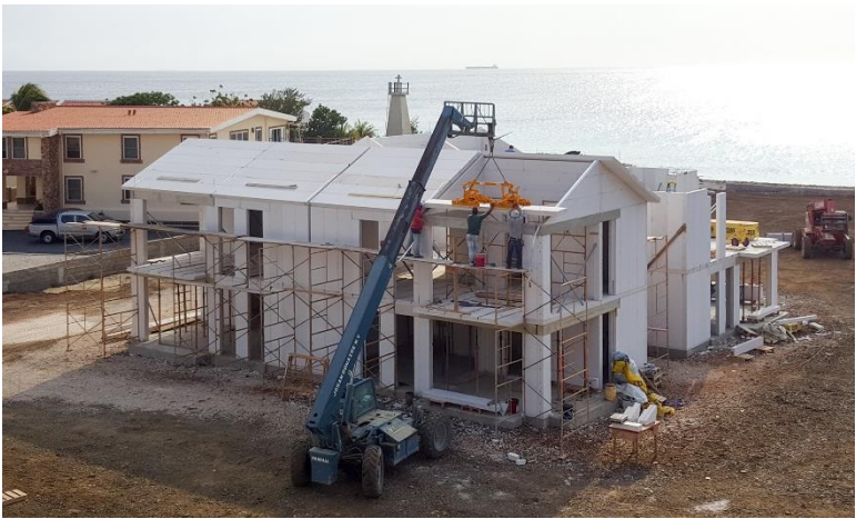
Installation of roof panels
