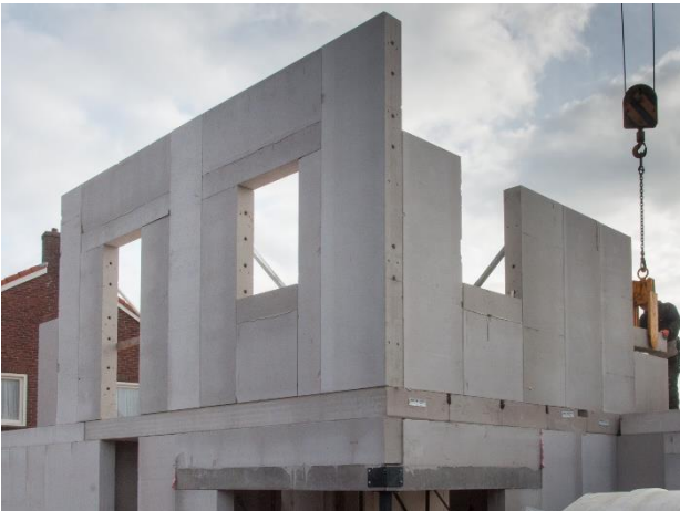
Installation of AAC wall panels
