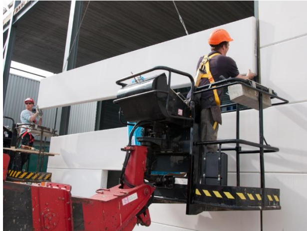
Installation of industrial wall panels
