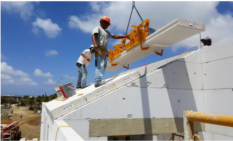
Installation of roof panels
