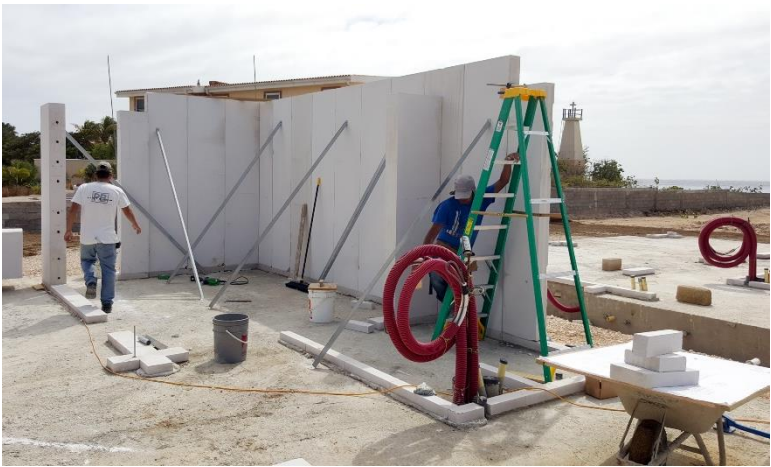
Installation of wall panels
