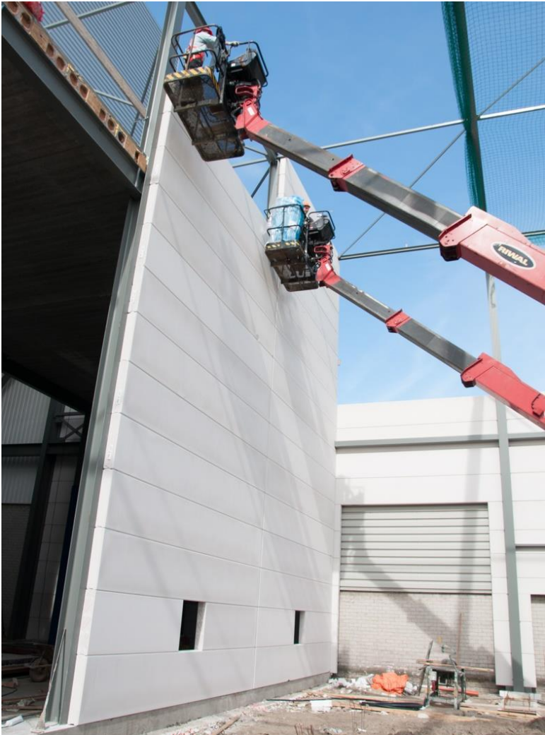
Installation of wall panels
