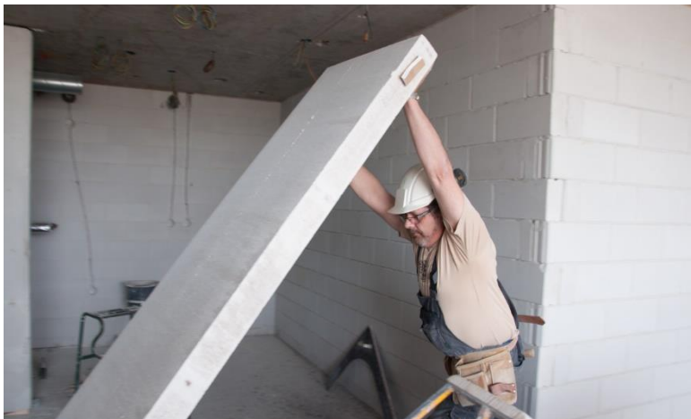
Push the panel in vertical position and move it in position
