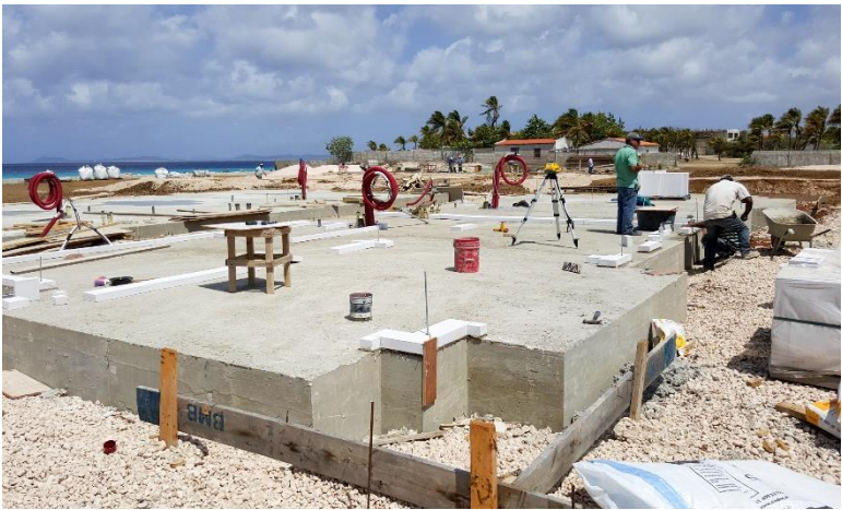
Installation of levelling blocks
