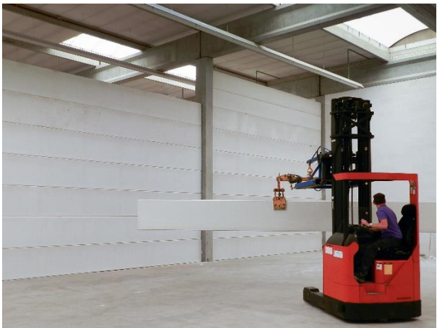
Installation of industrial wall panels
