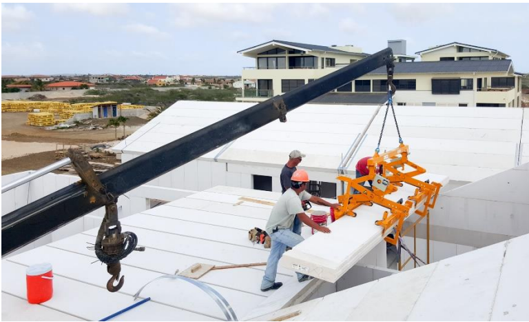
Installation of roof panels
