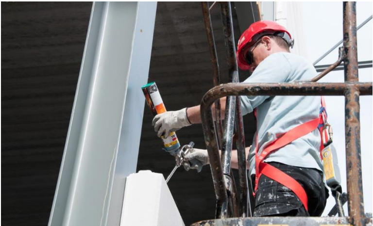
Fill up the anchor spaces with foam
