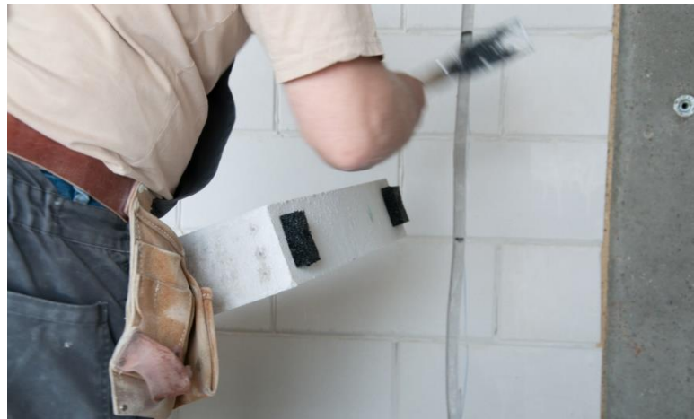
Place two rubber blocks on top of the panel, used for dialation
