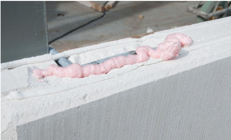
Anchor to attache the panel to the steel frame
