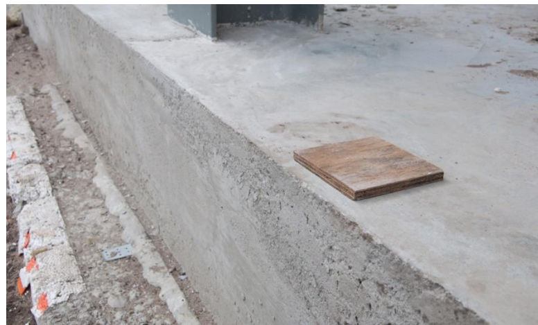
Placing level blocks
