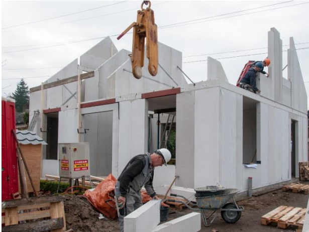
Building with the Aircrete Building System
