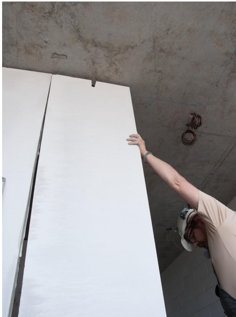
Align the panel with the previous panel(s) and the chalk line
