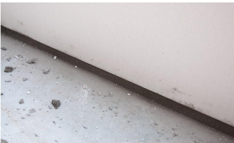
The space between the foundation and panel is filled with cement
