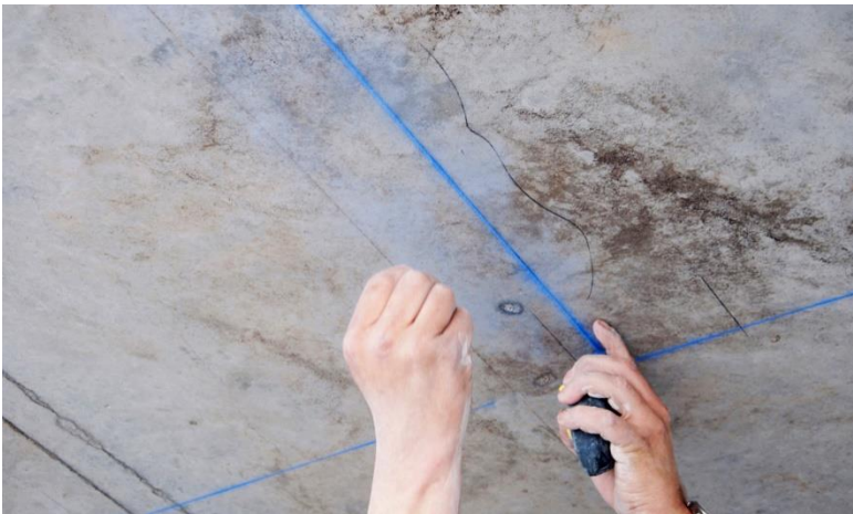
Draw the layout of the wall on the ceiling with a chalk line
