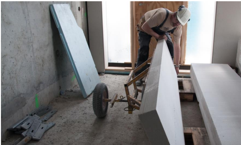
Use a panel lifting car to take the panels from the pallet
