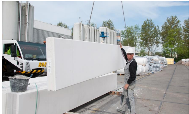
Transporting the panel by crane to installation
